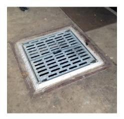
Steelway Bri-Grate is a mild steel lasered pull-through floor grid suitable for pedestrian duty traffic. We can fabricate from sizes of 300 x 300mm up to 1000 x 1000mm. All grids are galvanized to BSEN ISO1461.
